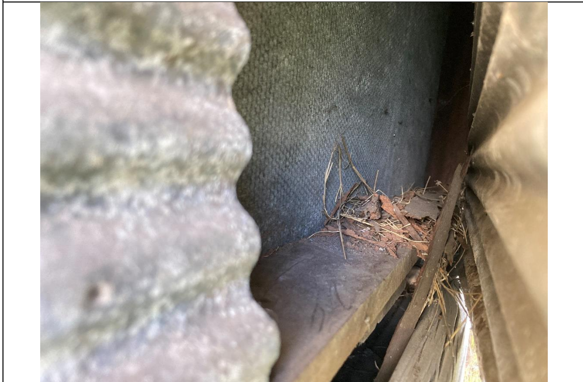
Photo 18: A view behind the cladding showing internal timber frame condition.
