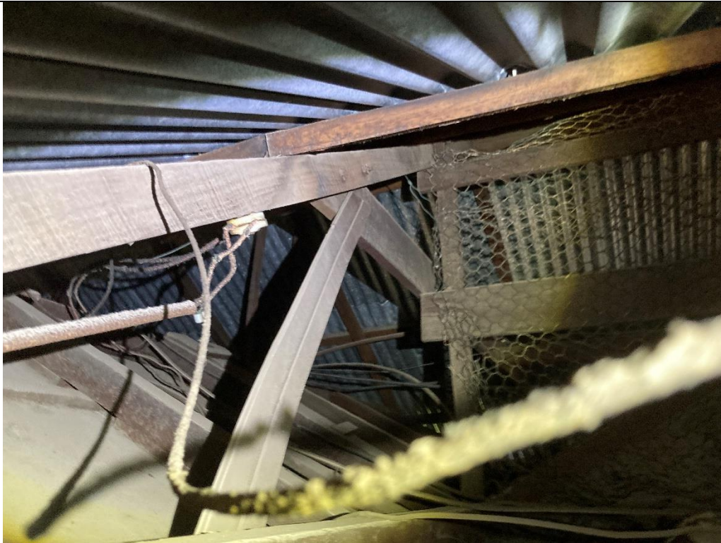
Photo 15: Overall view of roof members.
