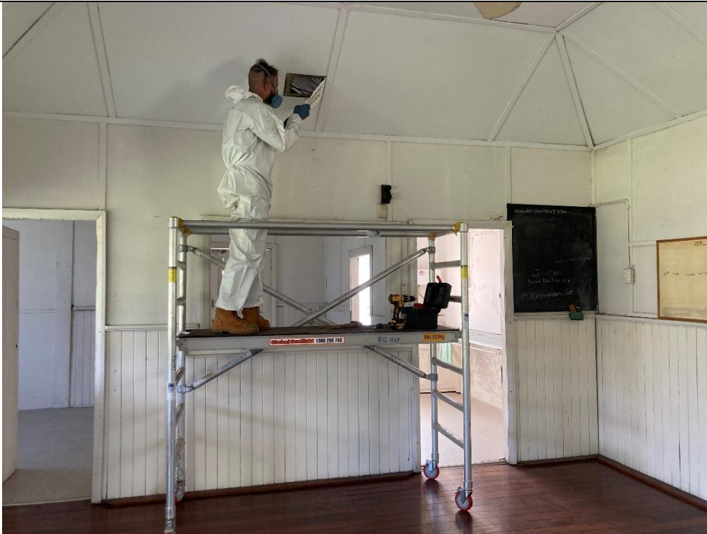
Photo 35: Set up the platform and carried out inspection through the air vent.
