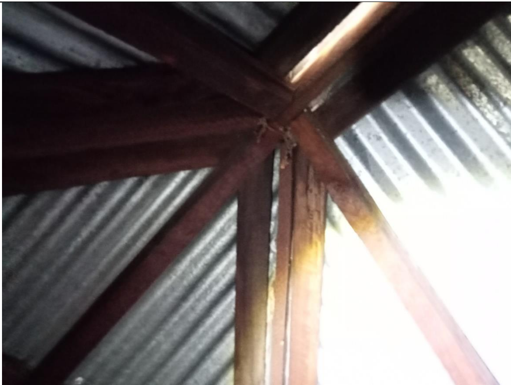
Photo 44: A close-up view of the roof framing work connection details.
