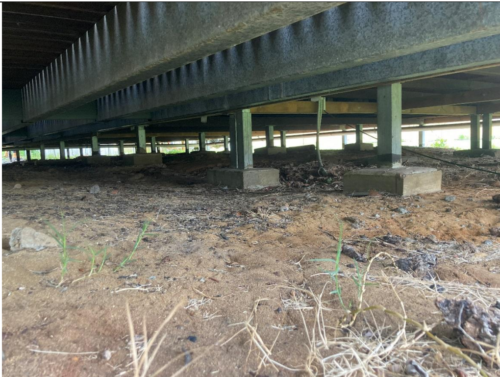
Photo 12: Overall view of floor beams and pad footings.
