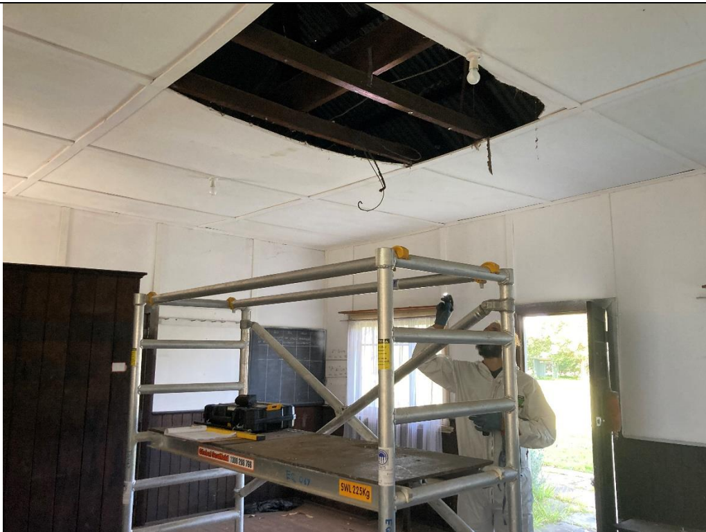
Photo 41: Set up the platform and carried out the inspection.
