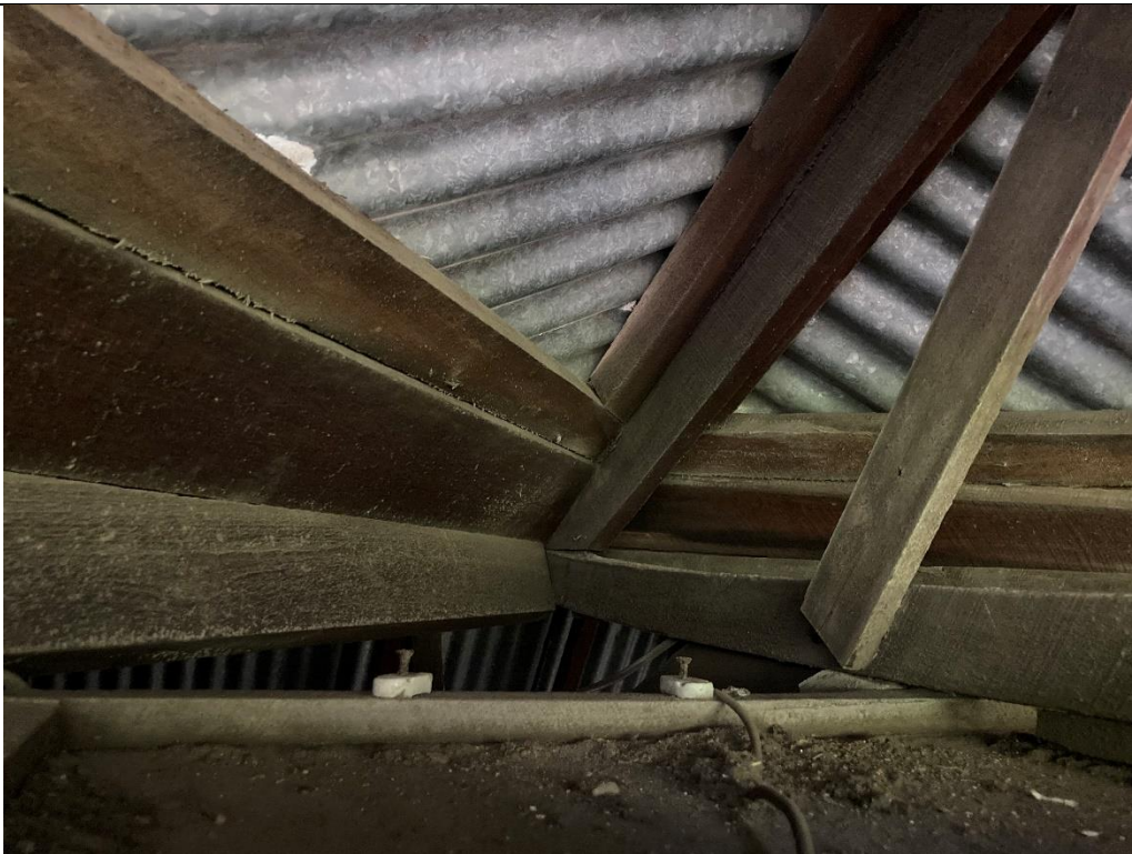
Photo 36: View of rafters beams.
