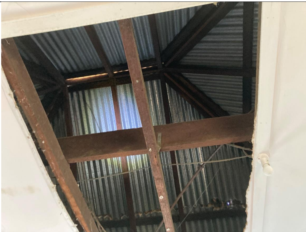
Photo 42: Overall view of the ridge beam and rafters.
