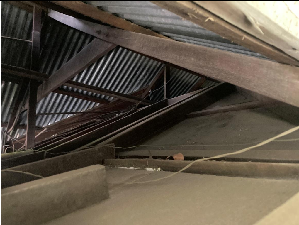
Photo 21: Rafter condition, looking southwest.
