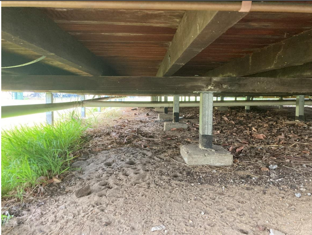
Photo 11: Overall view of pad footings.
